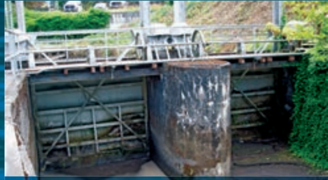
Headgates Remove and refurbish the headgates; replace motorized controls
