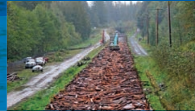
Timber Flume Replacement Replace 2,300 feet of 28 feet wide timber flume with 18 foot wide concrete flume; repair sections of existing concrete flume
