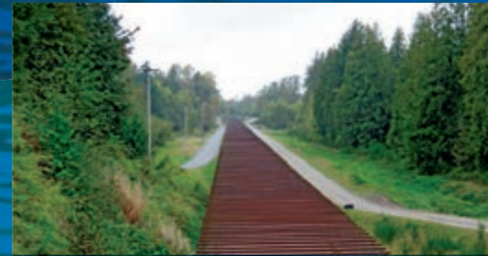
Timber Flume Replacement Replace 2,300 feet of 28 feet wide timber flume with 18 foot wide concrete flume; repair sections of existing concrete flume
