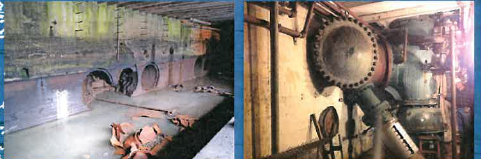
Powerhouse Inspected system; refurbished relief valves; repaired discharge tunnels.
