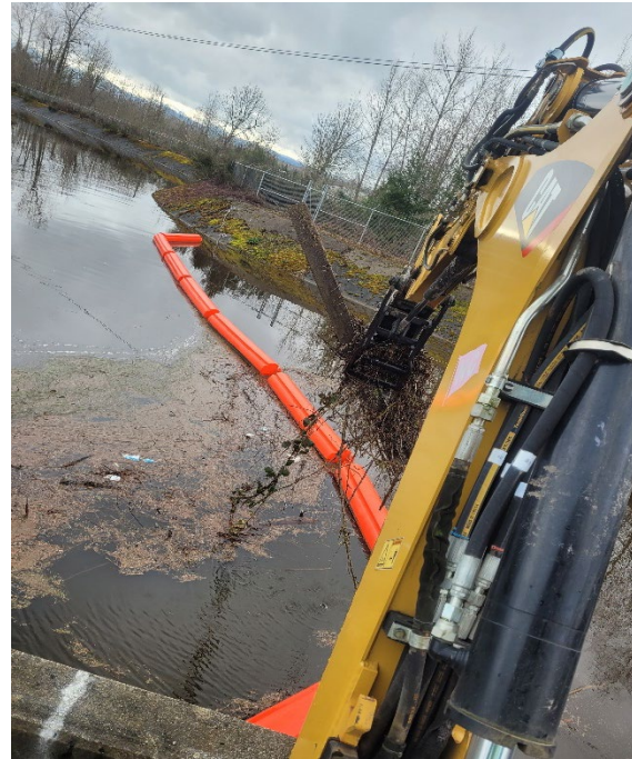
2. Pipeline Intake Log Boom Clearing By Twin Pipelines at 258 th Street.
