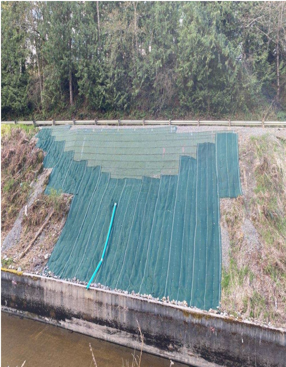
5. Fabric on the Slide Area.
