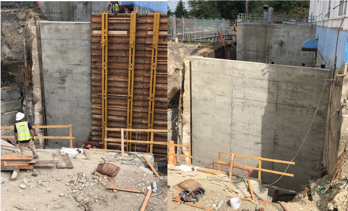
9/16/22 Retaining Wall forms removed, site prepared for backfill
