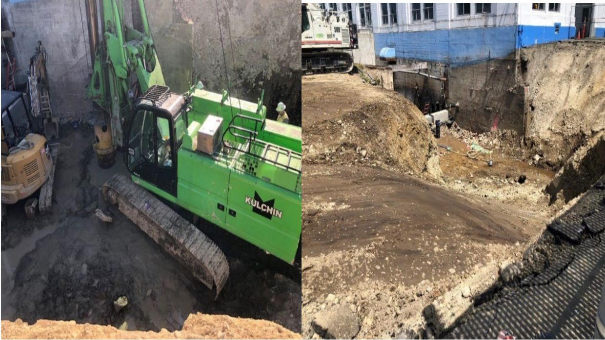
7/29/22 Excavation and Temporary Shoring Rig
