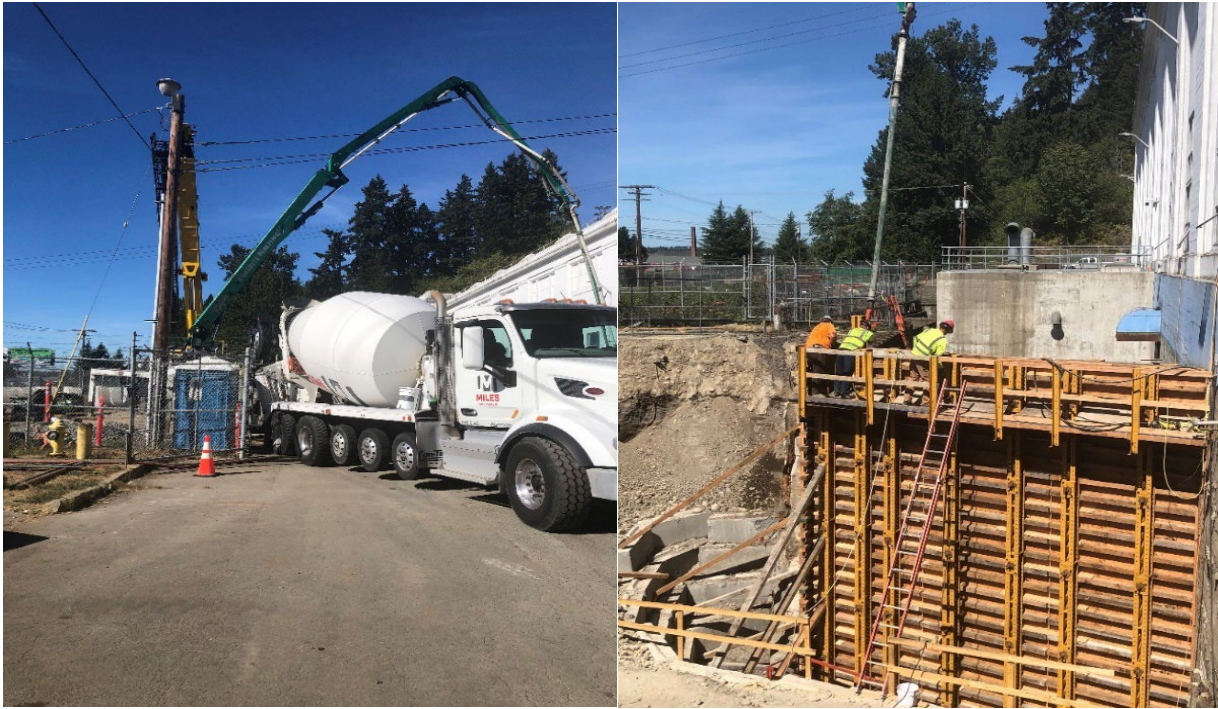
9/8/22 Retaining Wall Concrete Placed
