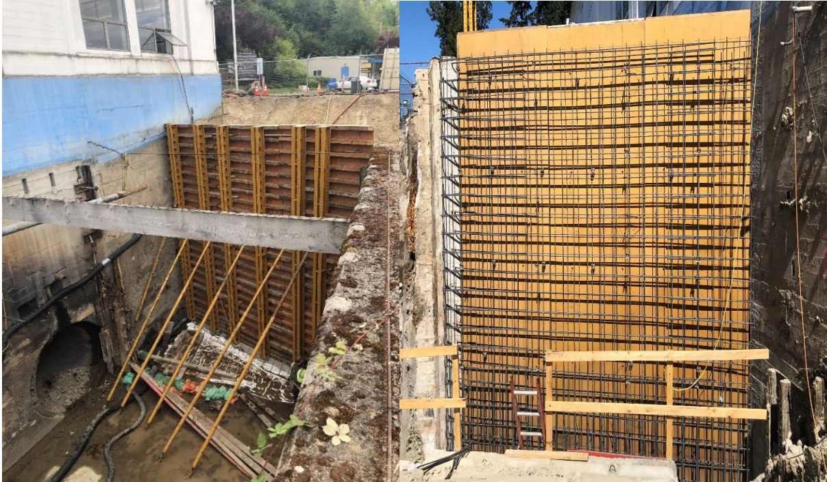
8/26/22 Retaining Wall Rebar Placement Wall Forming
