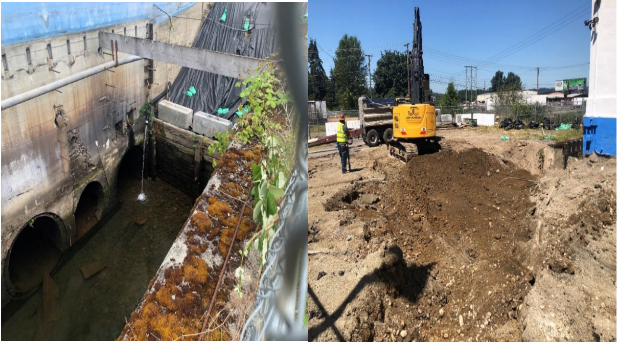
7/11/22 Construction Starts, Site Clearing and Excavation
