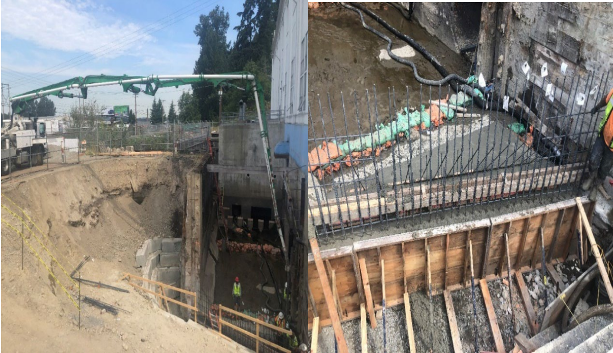
8/18/22 Concrete Placement Plunge Pool Floor and Retaining Wall Footing
