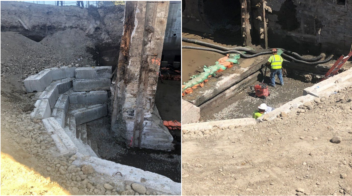
8/8/22 Footing and Plunge Pool Floor Forming
