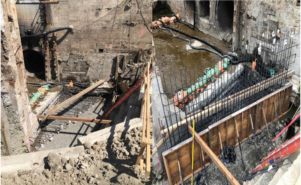
8/11/22 Rebar Placement for Plunge Pool Floor, Footing and Wall
