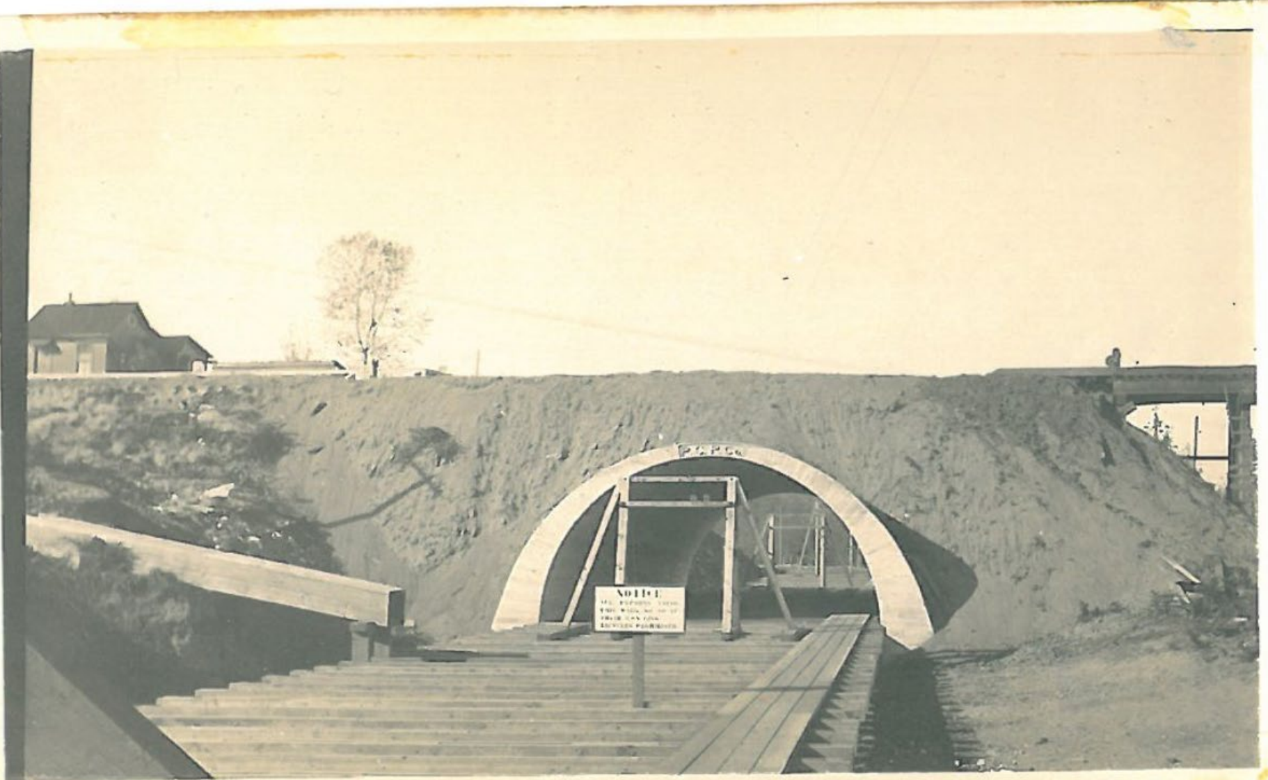
Flume going underneath the P&G Company Railroad, which is now a Rails-to-Trails walking path. Circa 2011
