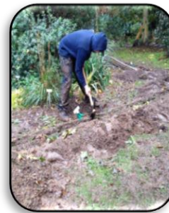
Learning how to install irrigation lines
