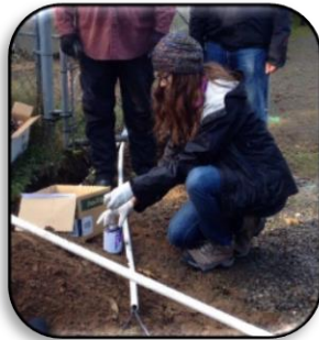
Learning how to glue irrigation lines
