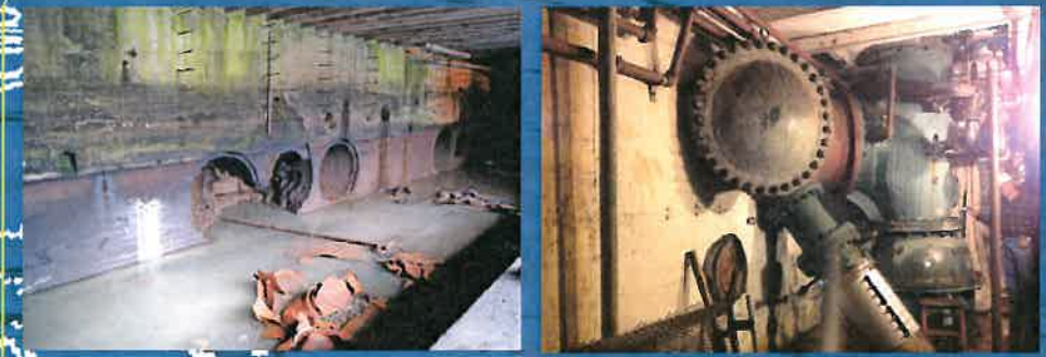
Powerhouse Inspected system; refurbished relief valves; repaired discharge tunnels.
