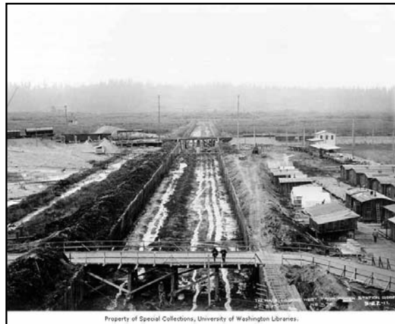
Tailrace west from powerhouse toward the White River, with view of main construction camp, September 22, 1911 (UW n.d.)
