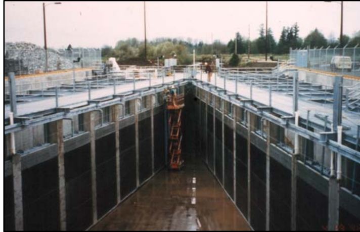
Fish screen (vee shape) for downstream-migrating fish Photo courtesy of R.C. Ladley, Puyallup Tribe Fisheries Division
