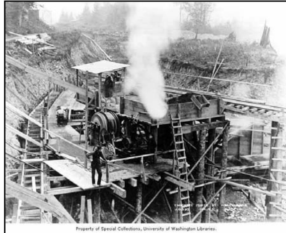
Concrete mixer at diversion dam headworks, September 15, 1910 (UW n.d.)
