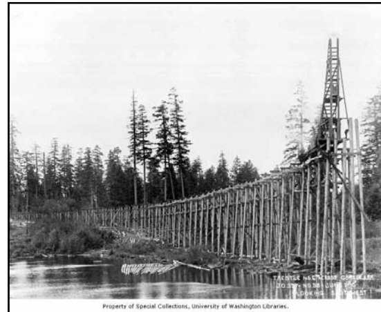
Construction of a railroad trestle across a northern arm of Lake Tapps, June 1, 1910 (UW n.d.)
