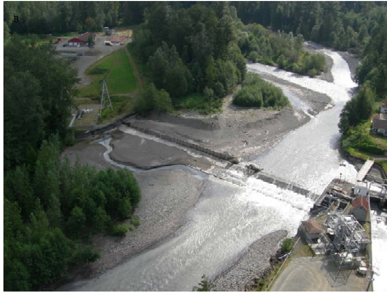
The diversion dam on the White River at RM 24.3. The fish ladder and trap and the intake to Lake Tapps Reservoir are at right. The fish hatchery operated by the Muckleshoot Indian Tribe is at upper left. Photo courtesy of R.C. Ladley, Puyallup Tribe Fisheries Division
