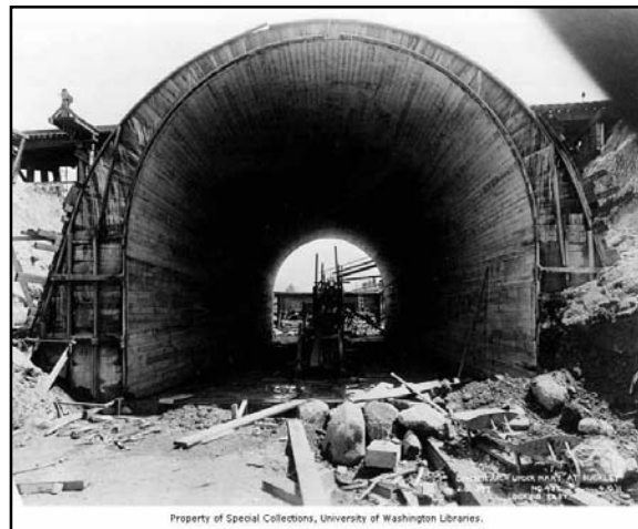
Concrete culvert for flume being built under railroad trestle at Buckley, June 10, 1911 (UW n.d.)
