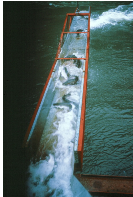
Fish ladder at the Buckley Fish Trap Photo courtesy of R.C. Ladley, Puyallup Tribe Fisheries Division
