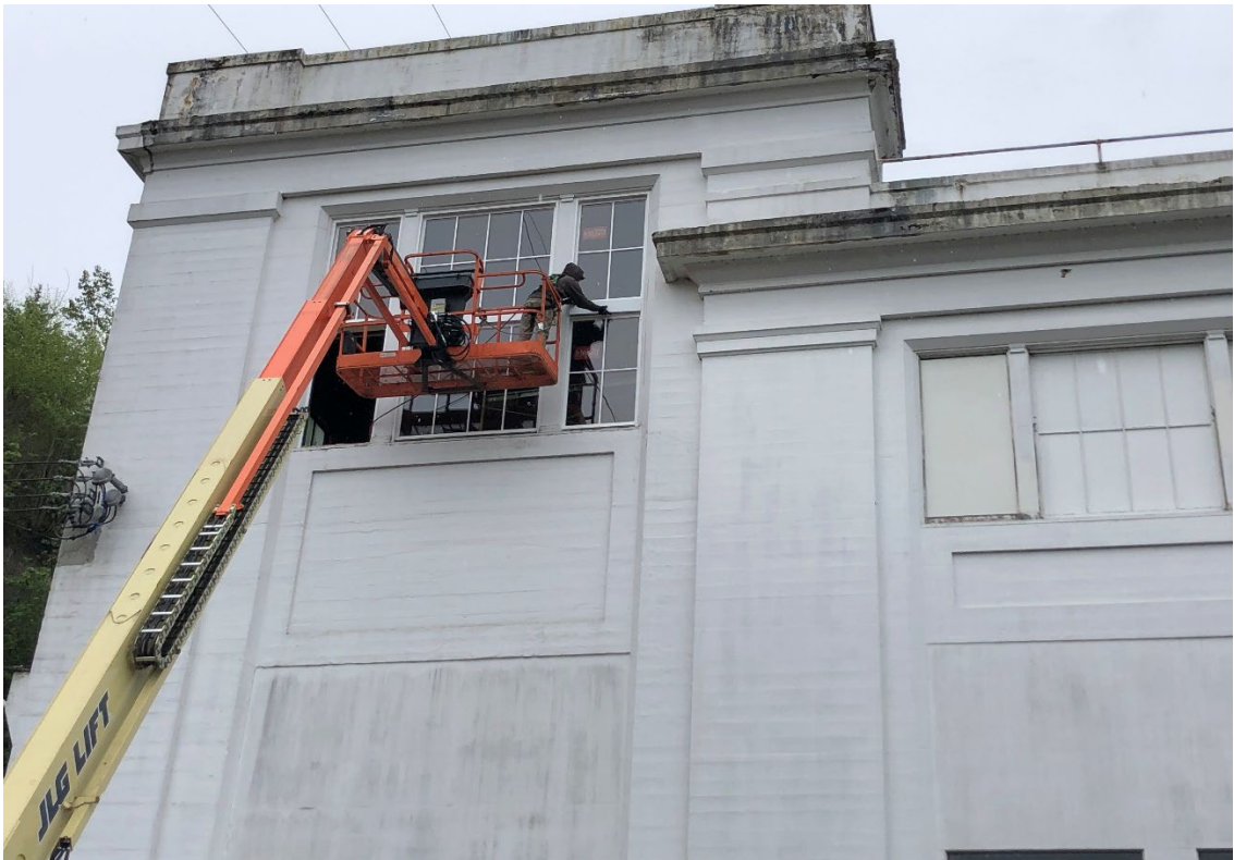
New Windows at the Powerhouse
