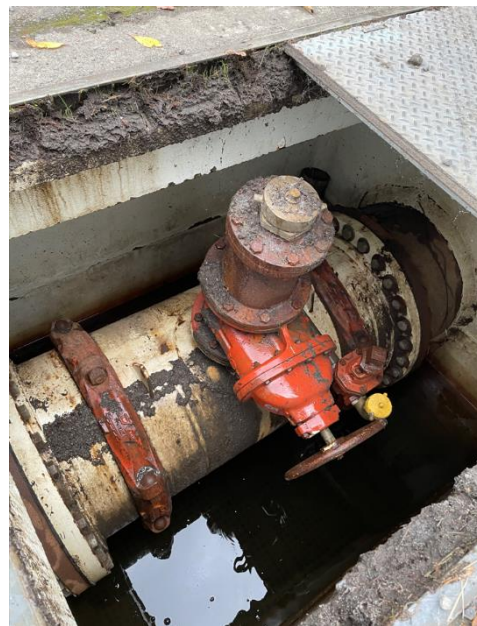
Bellevue-Issaquah Pipeline "pig station"
