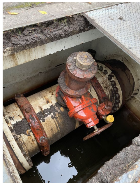
Bellevue-Issaquah Pipeline "pig station"
