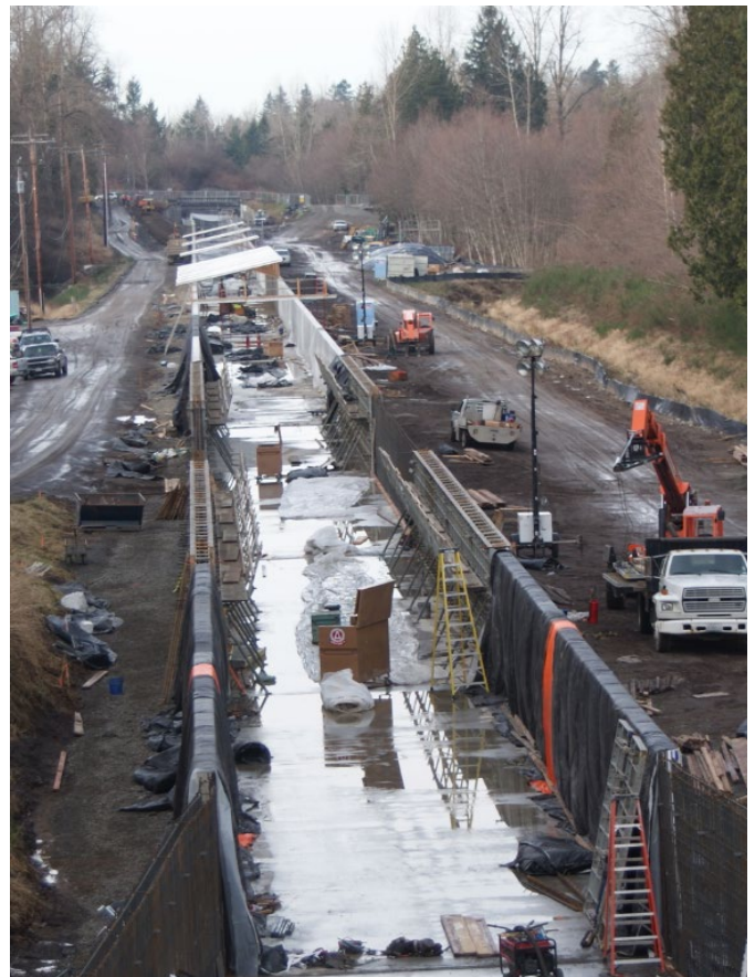
Replacing the wood flume with a concrete flume (2014)
