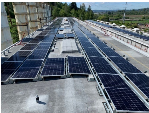
Solar panels installed on the Powerhouse in 2022.
