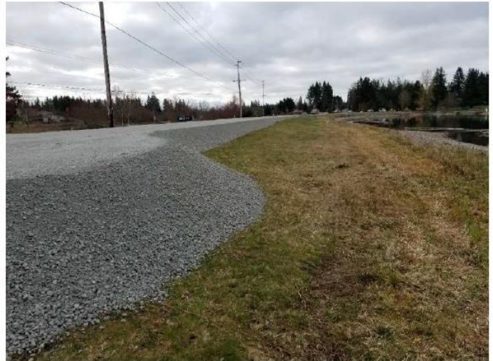
Dike 12 after raising
