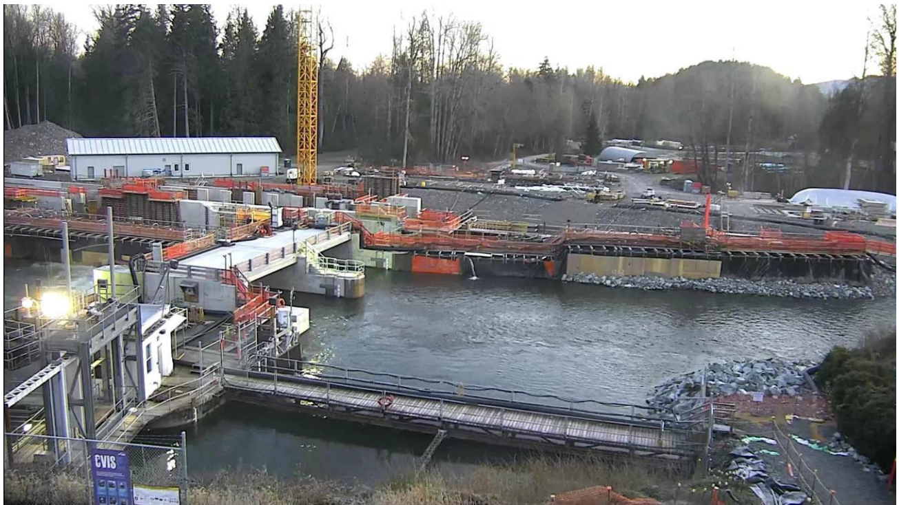
Construction of New USACE Barrier Structure – December 2020
