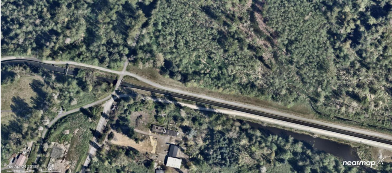
Aerial View of Flowline
