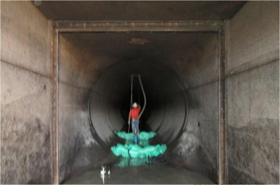
Interior of 12-Foot Tunnel
