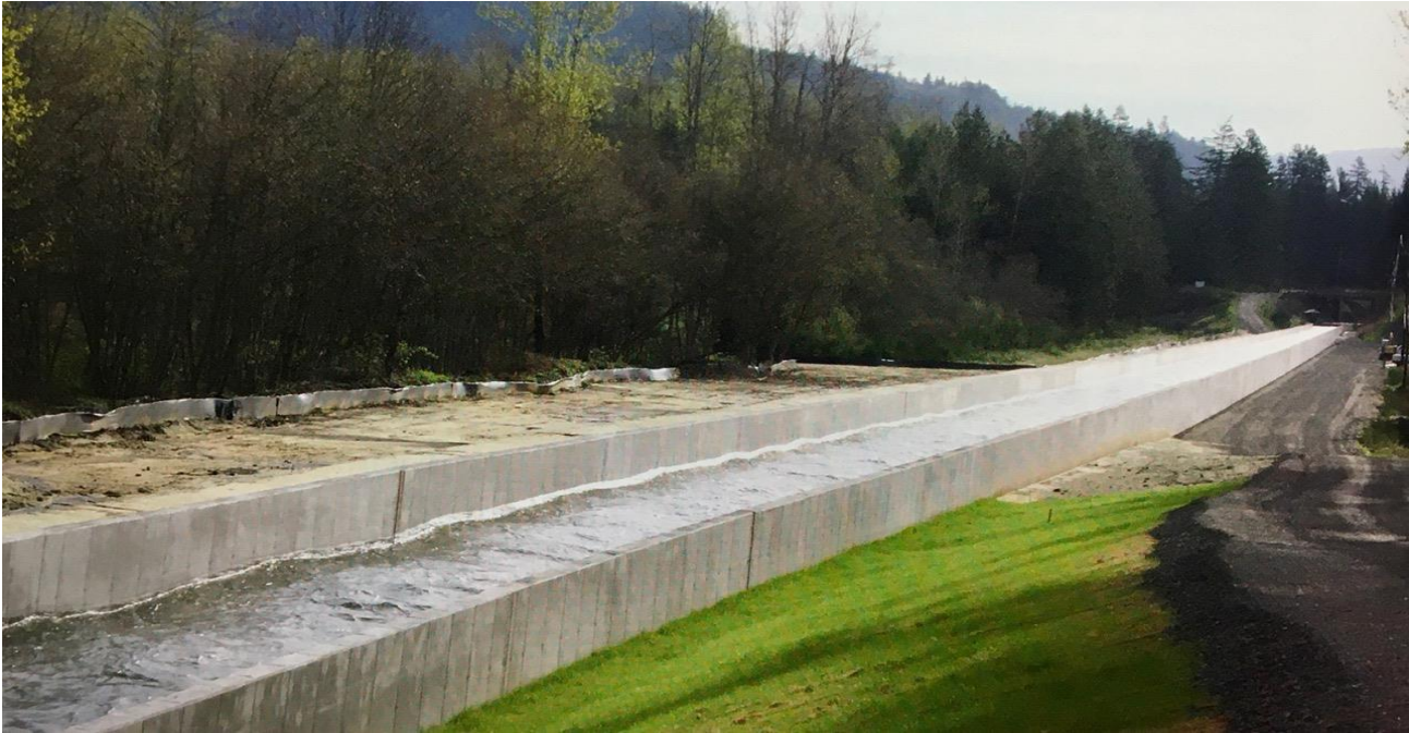
Concrete-Lined Canal Section of Flowline
