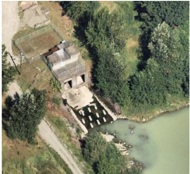
Outlet Structure (Valve House)
