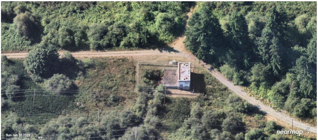
Aerial View of Forebay
