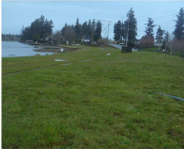
Dike 12 before raising
