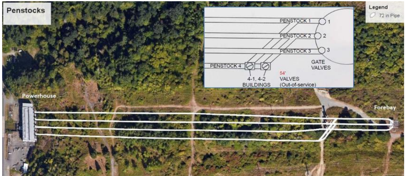
Aerial View of Penstocks and Standpipes
