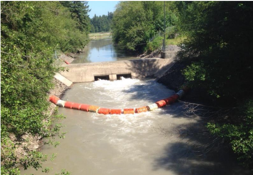
Debris boom at Backflow Preventer Facility
