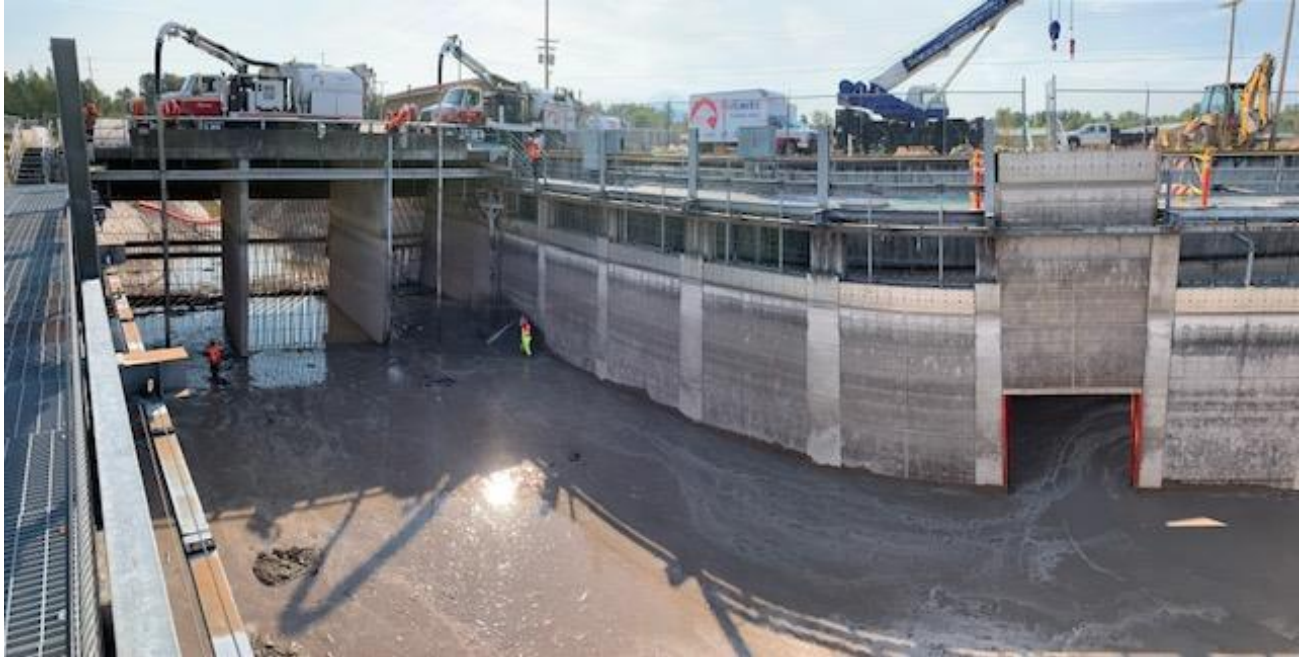
Cleaning and Sediment Removal at Fish Screen Facility – September 2021
