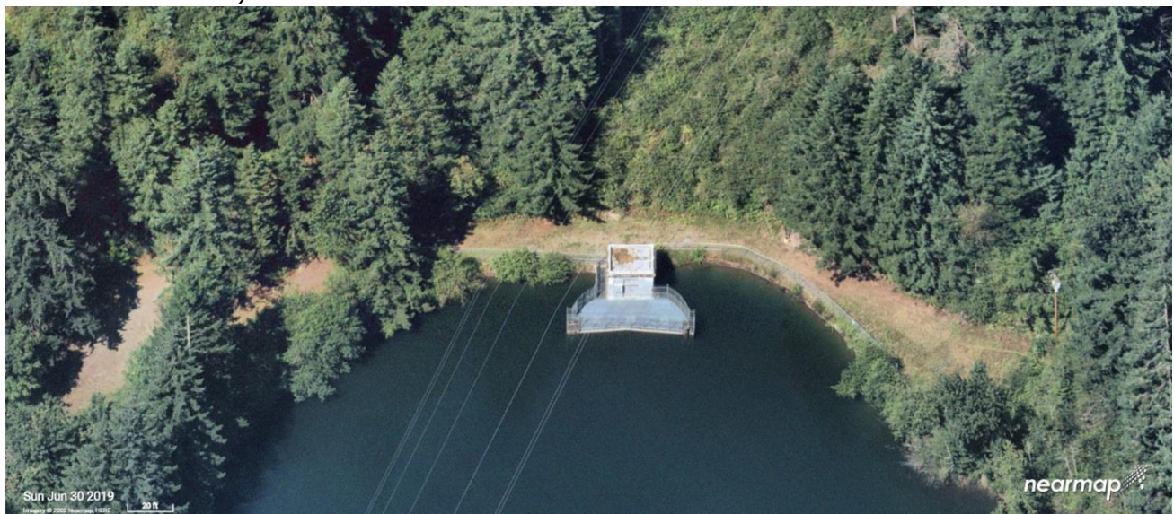
Tunnel Intake Facility
