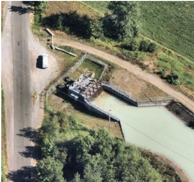
Intake Structure and Trash Rack
