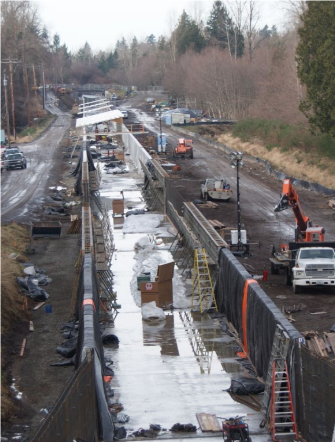
Replacing the wood flume with a concrete flume (2014)
