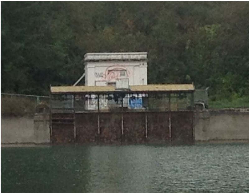
Tunnel Intake facility
