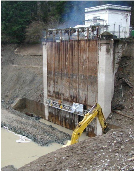
Old Tunnel Intake trash rack
