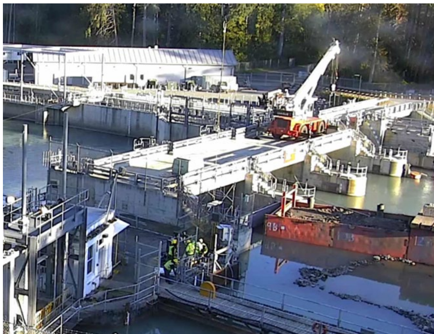
Headworks Intake Modifications Project
