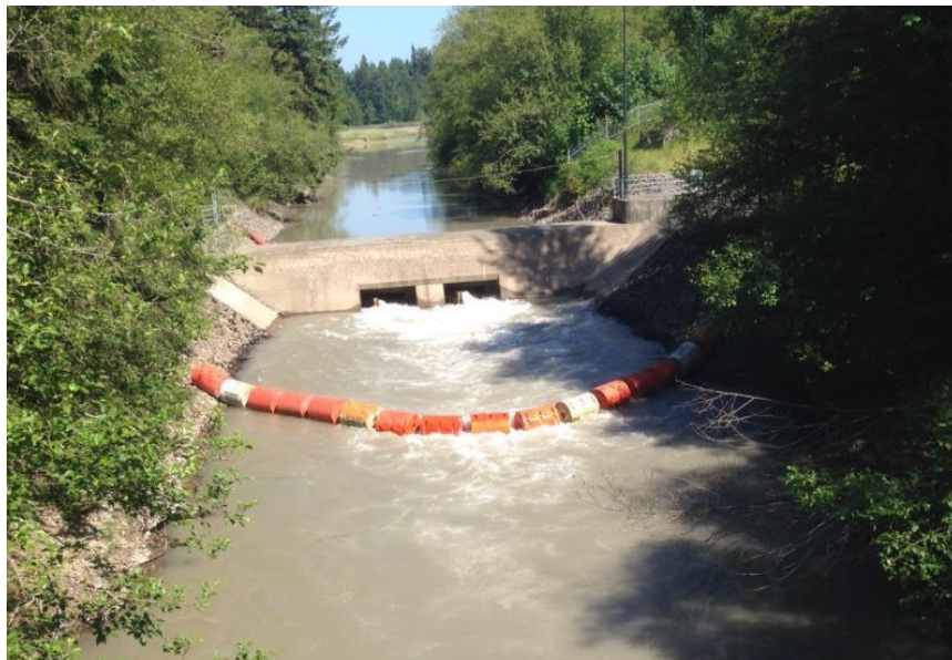
Debris boom at Backflow Preventer Facility
