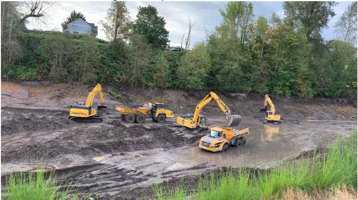
Sediment Removal at Wolslegal Basin – September 2021
