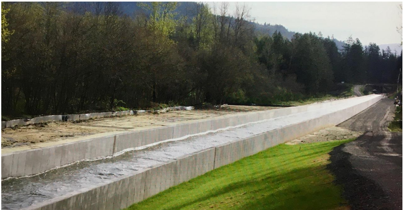
Concrete-Lined Canal Section of Flowline
