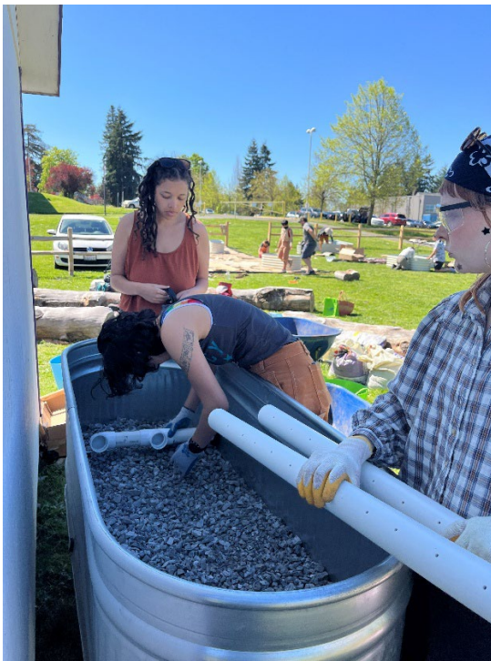
Soil and Water Stewards Install a Rain Garden
