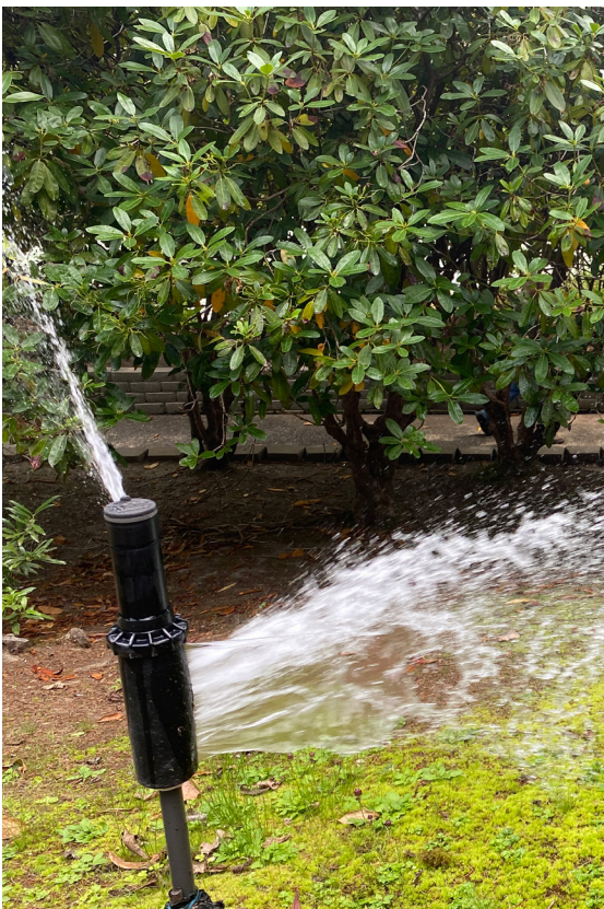
Breaks and leaks waste water and stress thirsty plants
